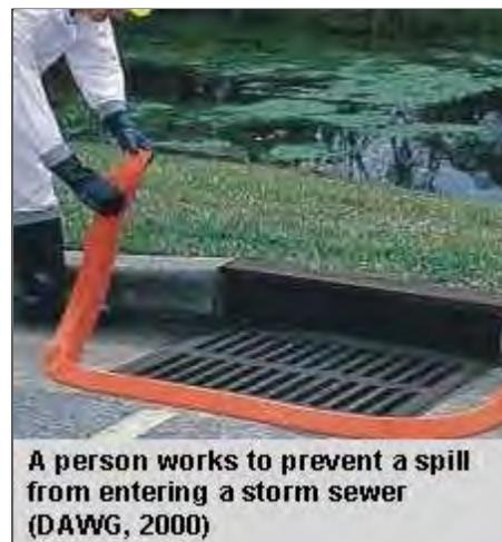
A person works to prevent a spill from entering a storm sewer (DAWG, 2000)
